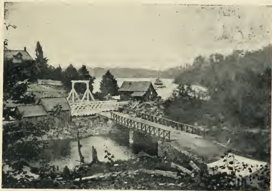
PORT CARLING, SHOWING LOCK AND MINNEHAHA BAY.
